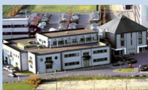
Site Maintenance GOSSELIES
